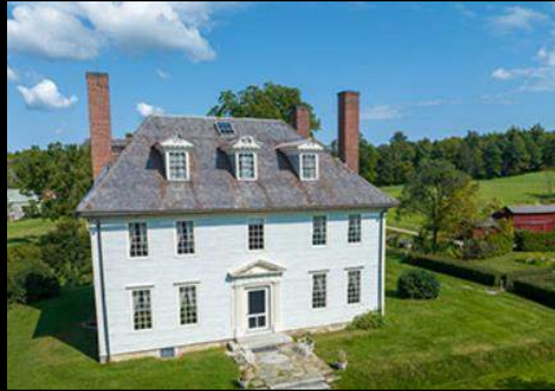
Hamilton House, South Berwick, MA 1785
