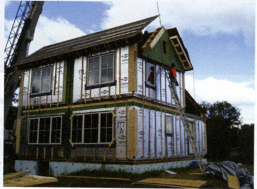
Building Blocks The modular boxes that make up the ART House are placed on the foundation, and then its roof panels are assembled.
