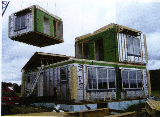
Building Blocks The modular boxes that make up the ART House are placed on the foundation, and then its roof panels are assembled.
