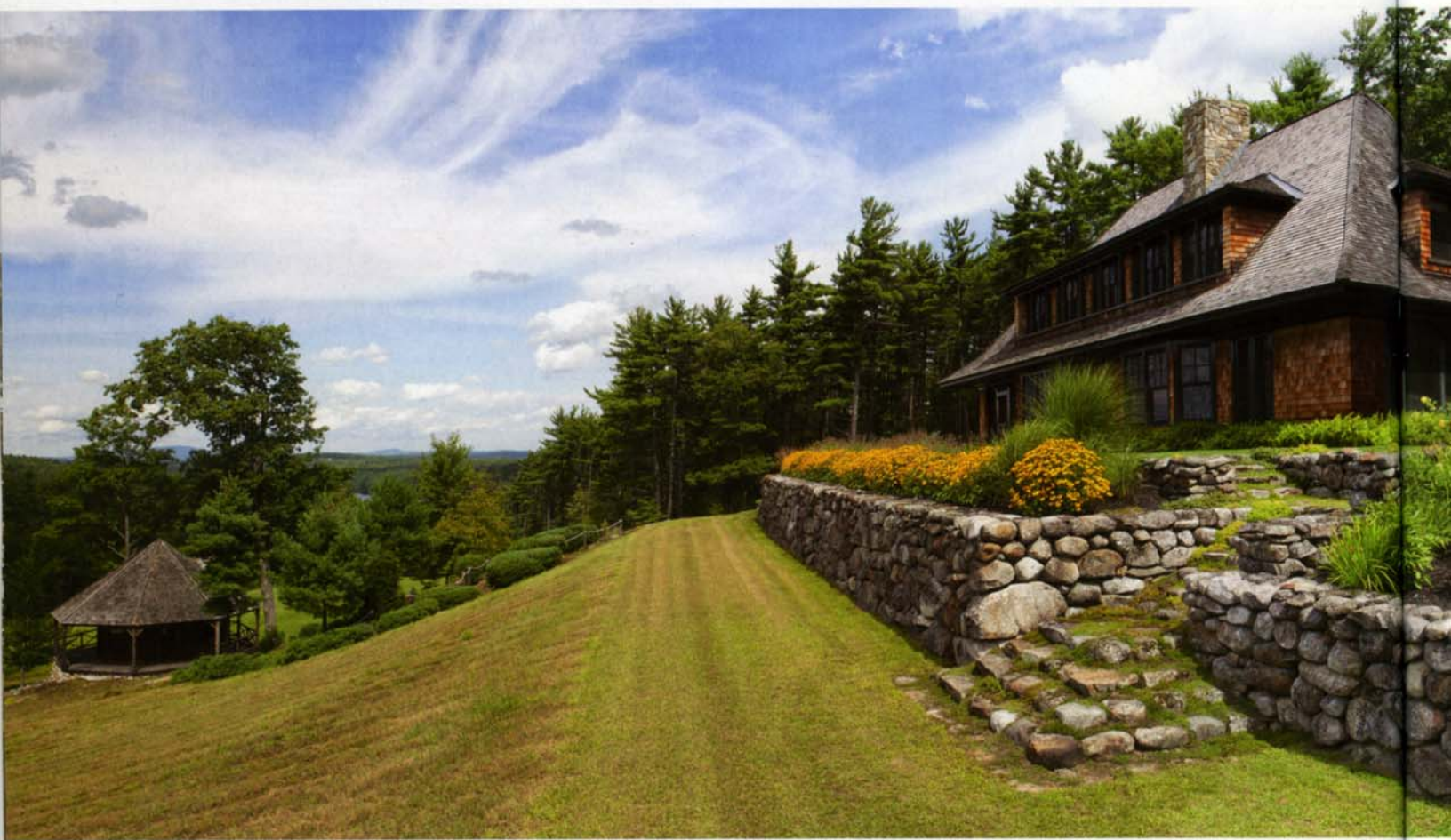
The hand-built stone retaining walls blend in with older stone walls on the property.
