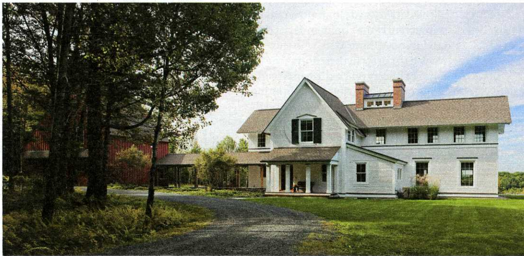
FITTING RIGHT IN From the front, the white clapboard structure looks like it belongs to Vermont.
