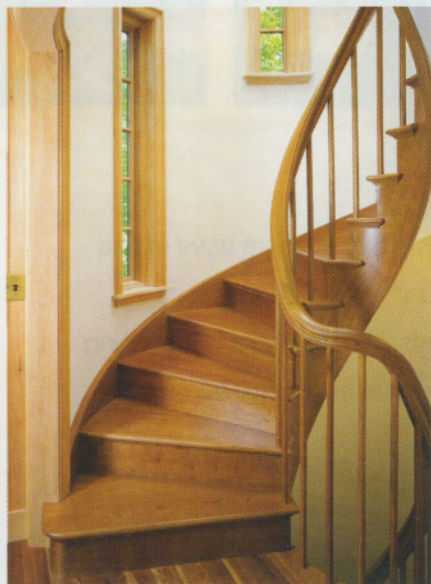
The second-floor bedroom has low eaves and a horizontal band of small windows wrapping around the east and south sides. BELOW: The circular stair was built without a center post.
