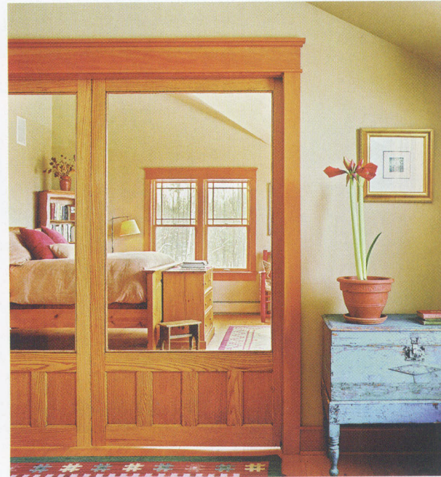
Looking back through time. Salvaged antique doors are given a starring role separating this anteroom from the master bedroom. The simple Arts and Crafts-style Douglas-fir casing allows the oak doors to take center stage. Designer: Heidi Arnold. Builder: Gristmill Builders, Stowe, Vt. Photo by Susan Teare.
