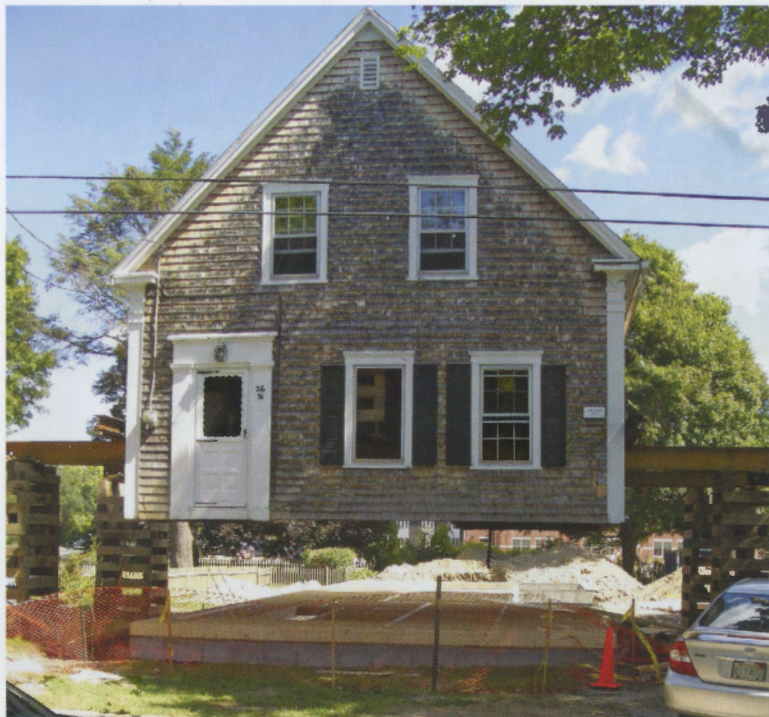
A problematic foundation below the existing cottage needed complete replacement. The solution was to lift the house on massive steel girders (needles) and build under it (left). Once replaced, it regained its Greek Revival elegance (above). (Courtesy of Albert, Righter & Tittmann Architects.)
